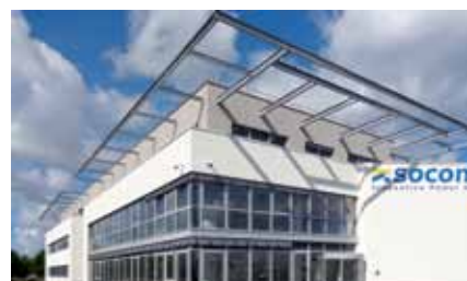
Socomec Green Building.
