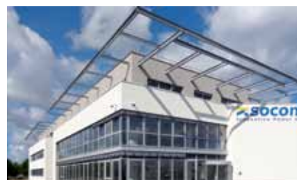
Socomec Green Building.
