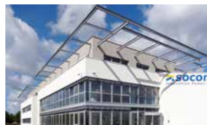
Socomec Green Building.
