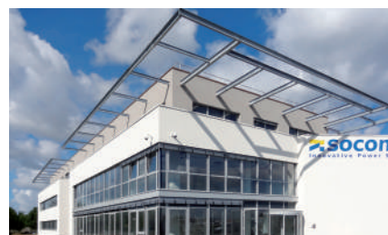
Socomec Green Building.
